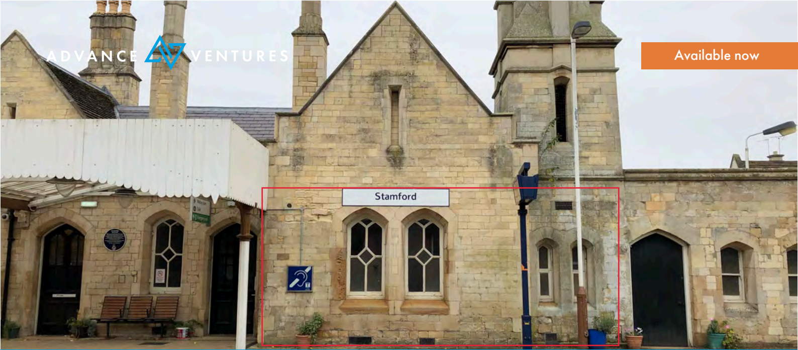
Retail Unit - Stamford station
